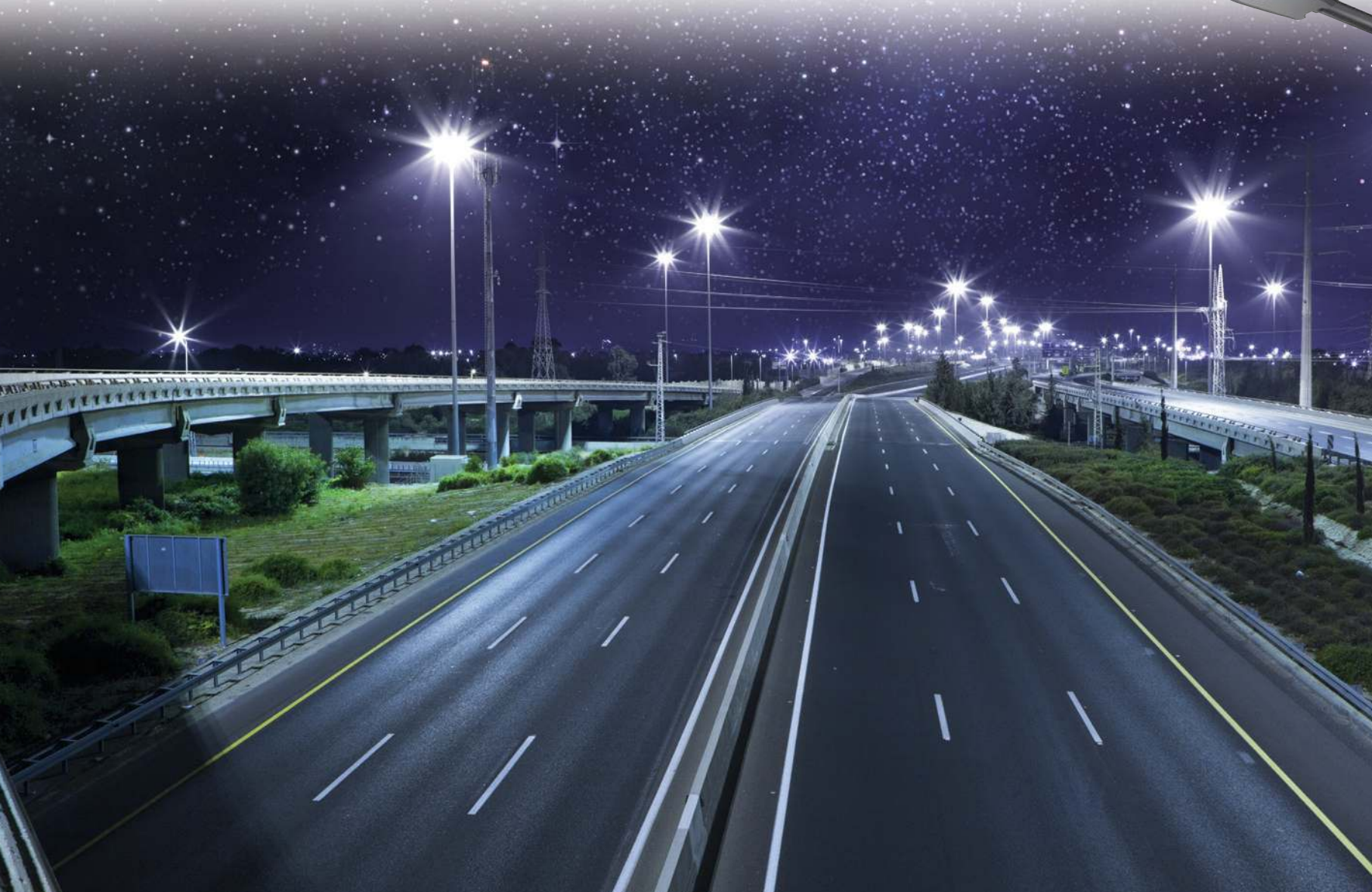
STREET LIGHT 90W
